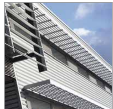
SUNCLIPS' & ICARUS' RENSON HQ, Waregem (BE) Arq.: Jo Crepain, foto: Nikke Bourgeois
