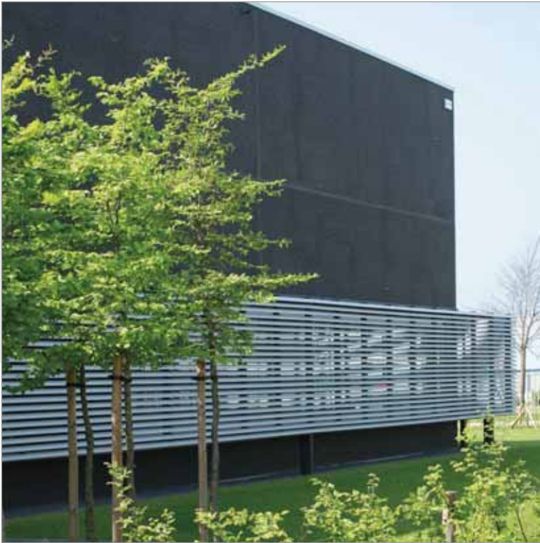
Play - De Pijpela's, Deinze (BE) - arq.: Engineering office Maes P, Marke
