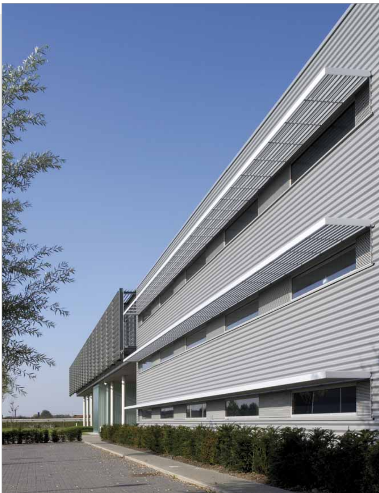
RENSON, Waregem (B), arq.: j. Crepain • foto: Toon Grobet
