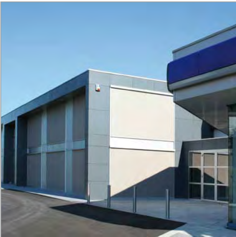
Volvo Garage Diksmuide, Architect Steraan Hoet
