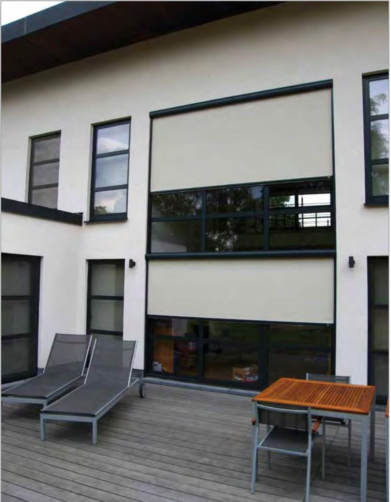
Installation by Meeussen (horren.be)
