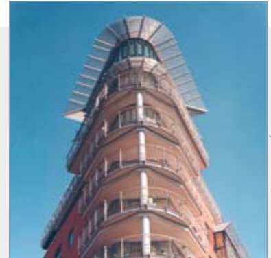
King Edwards Wharf, Birmingham (UK) arch.: Ian Darby Partnership
