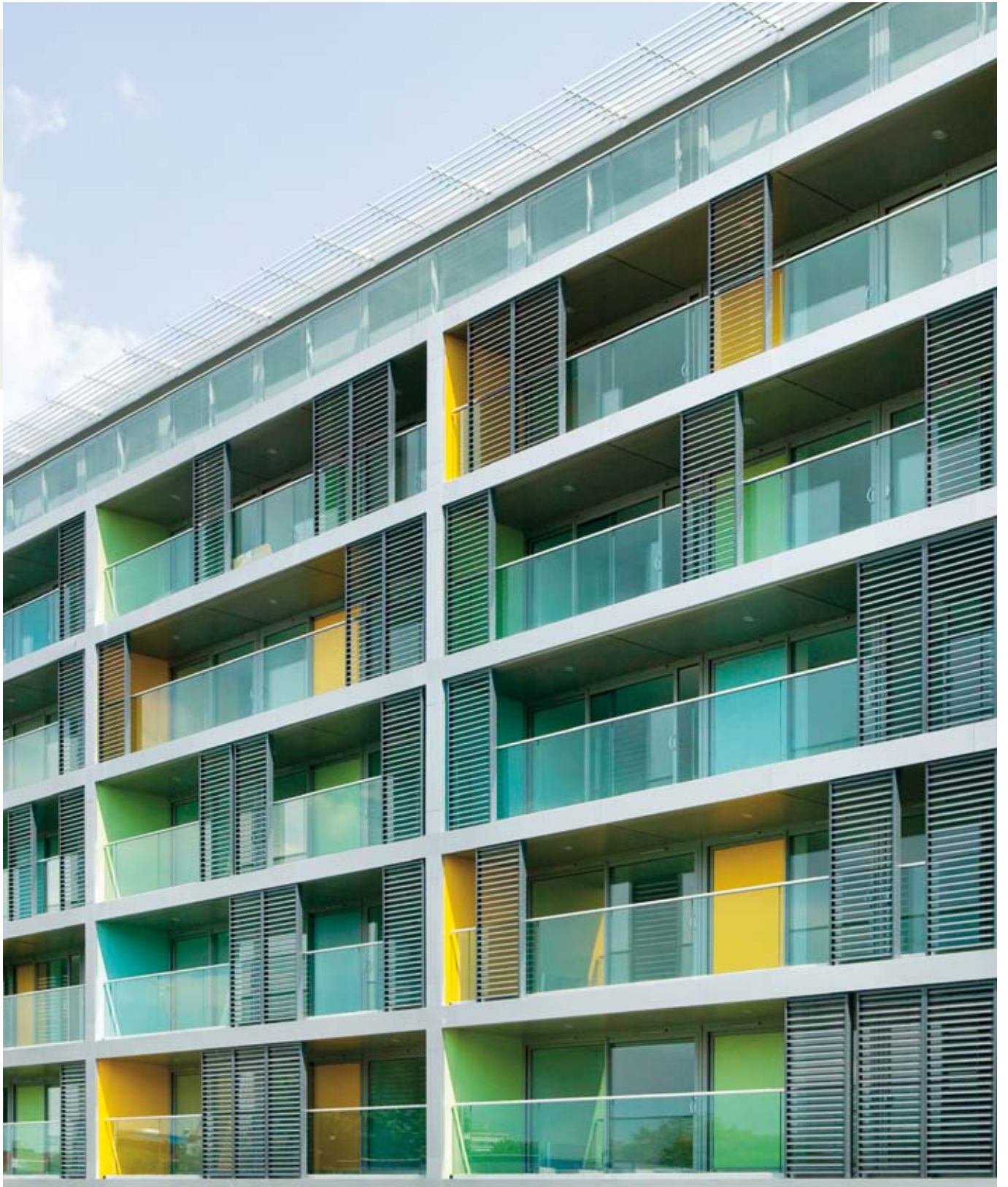
Ref. : Candy Wharf, Copperfield Road – London (UK), SUNCLIPS® Patio Evo 96
